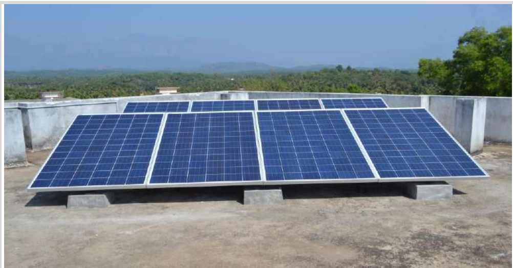
2 kWP SOLAR PHOTOVOLTAIC PLANT
