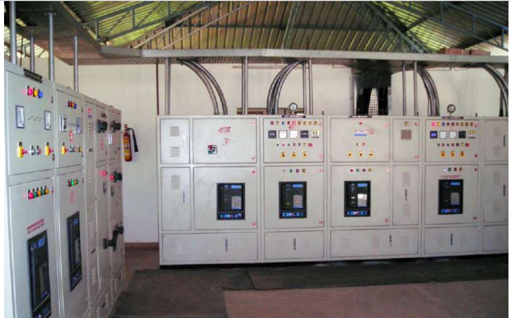
POWER HOUSE CONTROL PANELS 300kVA and 300kVA generators
