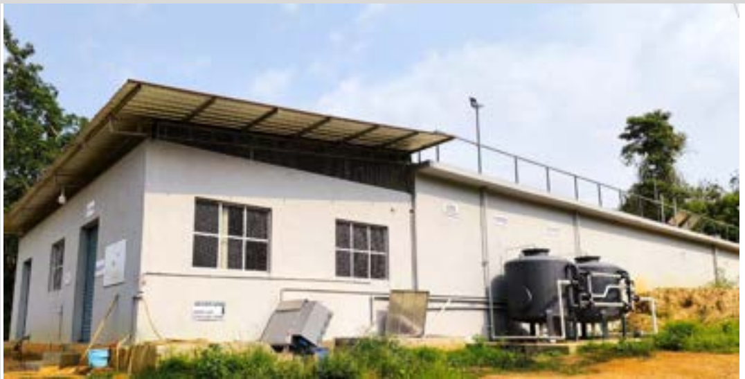
Two Sewage Treatment Plants (STP)
