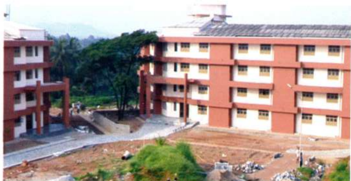
View of the New Hostel Blocks
