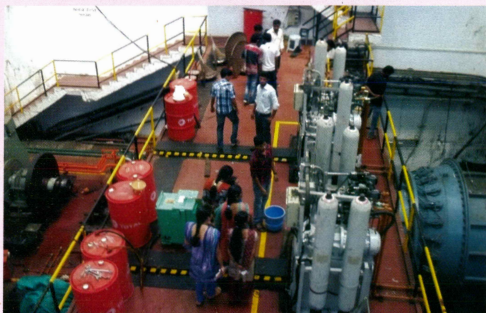
Students of 6th semester EEE Visited Bhoruka Hydel Power Plant
